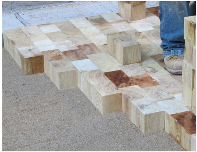
Black Locust installation over sand, no grooves, no mesh.
