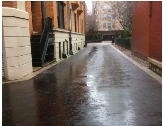
Black locust pavers street application wet from rain.
