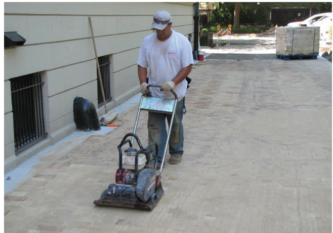
Vibrating sand joint filling.
