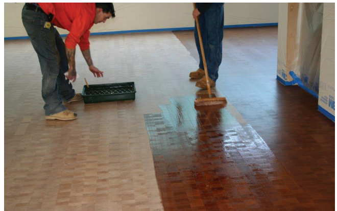
Applying Woca Oil using lambswool applicator
