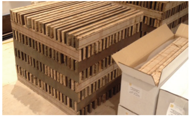
Open stack acclimation of prefinished strip blocks
