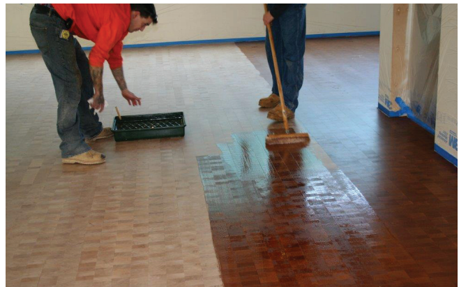
Applying Woca Oil using lambswool applicator
