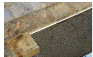
1 1/2 " depth x 4" x 4" Black Locust on gravel with, aluminum spine connection
