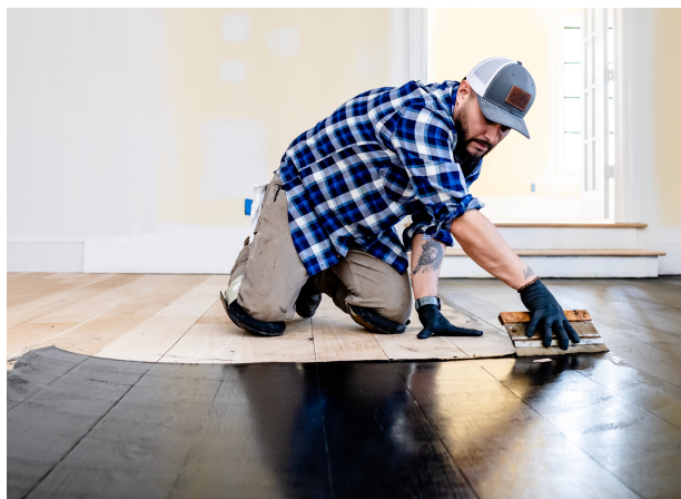
Applying UnoCoat® using the trowel method.
