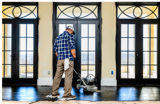
Removing excess UnoCoat® with a standard buffer and white pad.
