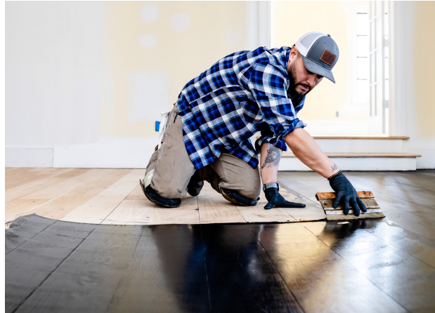
Applying UnoCoat® using the trowel method.
