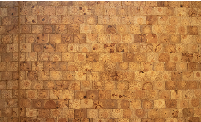
Pivot Centre (close up), Cleveland Ohio Southern Yellow Pine Blocks, sanded, finished with A106 Clear Sealer, w/cork expansion joint on the left side
