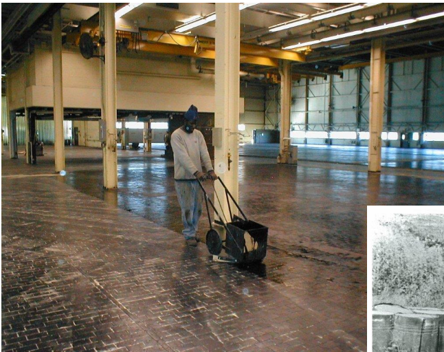
Squeegee Machine application of A-106 Black Sealer
