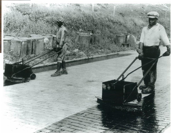
Squeegee Machine application of hot coal tar pitch on a wood block street, circa 1900
