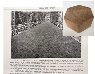
1 1/2 " depth x 4" x 4" Black Locust on gravel, with aluminum spine connection
