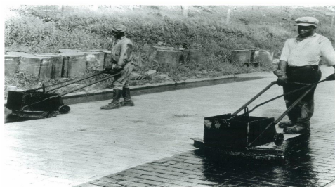
Squeegee Machine application of hot coal tar pitch on a wood block street, circa 1900
