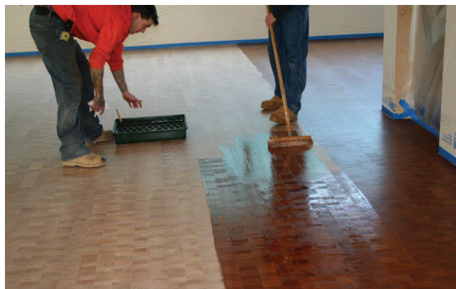
Applying Woca Oil using lambswool applicator
